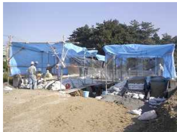
Figure - 4 Overall view of experiment equipment
